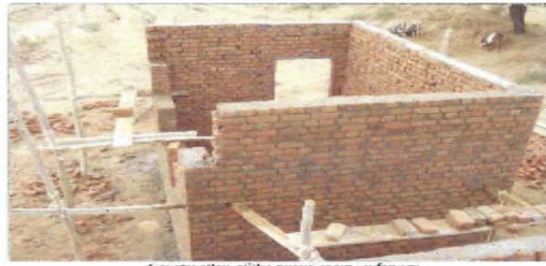
Construction of the main room under construction
