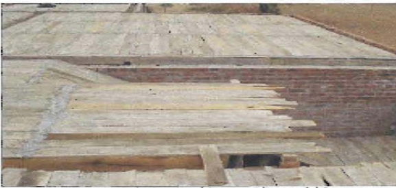
Preparation for pouring of the ground floor roof slab
