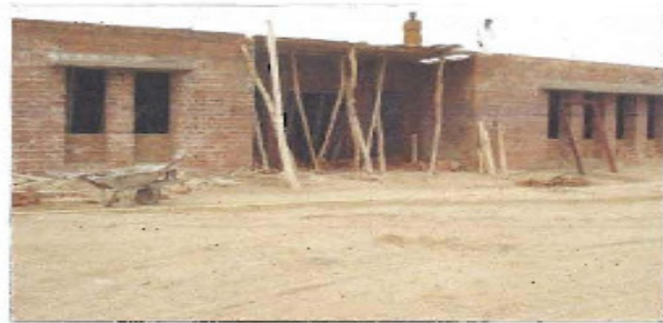
Exterior view from side of the under construction campus
