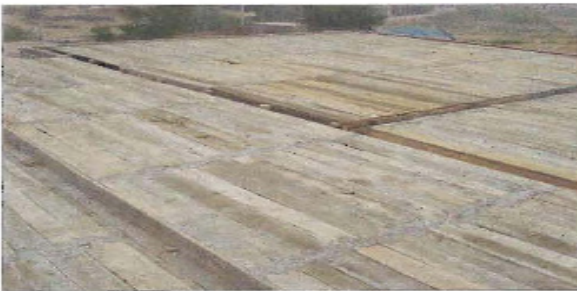
Preparation for pouring of the ground floor roof slab
