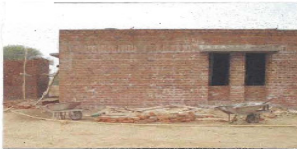
Construction work in progress of the side
